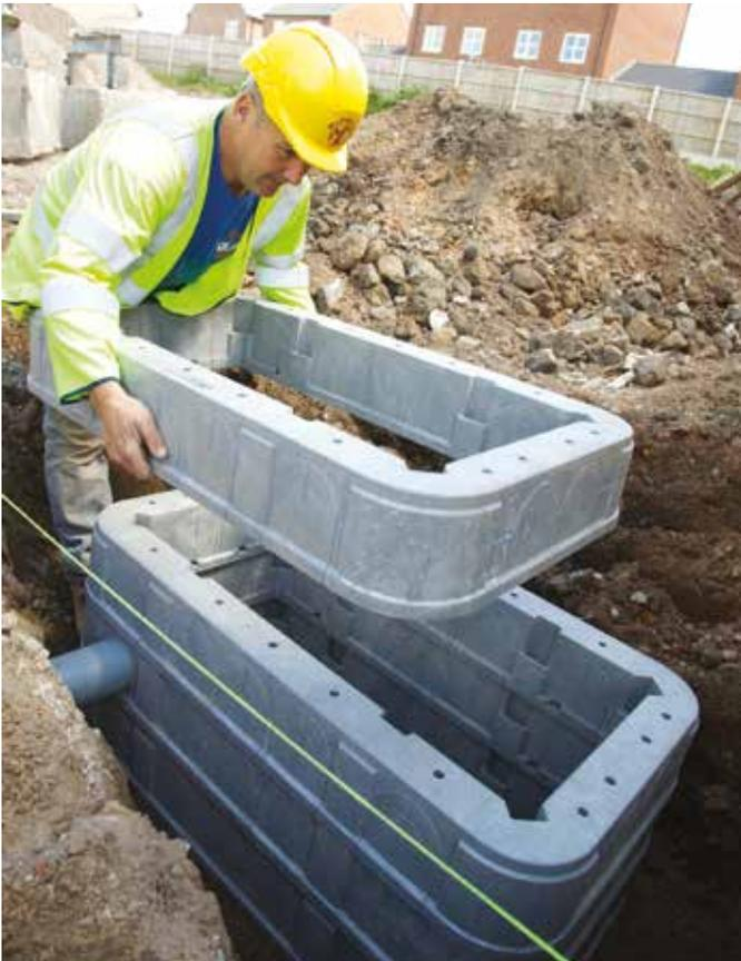
Box furniture items slot into moulded pockets within the chamber, eliminating the need to cast-in fixings or drill on site. Duct entries are also easy to achieve, using a standard hole saw mounted on a cordless drill.
