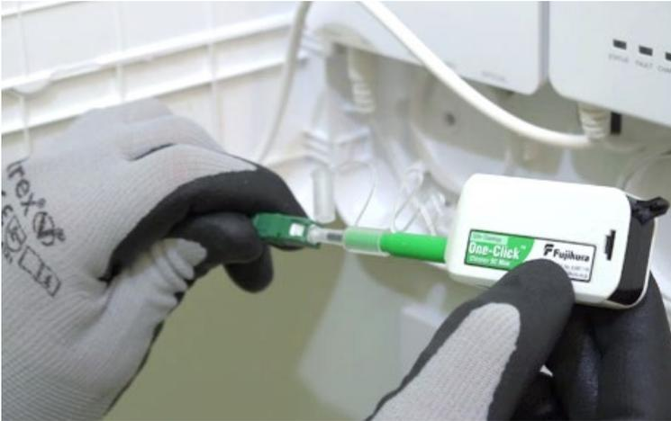
Remove the cap from the green fibre connector and use the One Click cleaner to clean both the connector and the optical port on the ONT. Once cleaned plug into the Optical port on the ONT. Care must be taken at this stage not to contaminate the end of the fibre connector to avoid any dirt from inhibiting the data signal.
