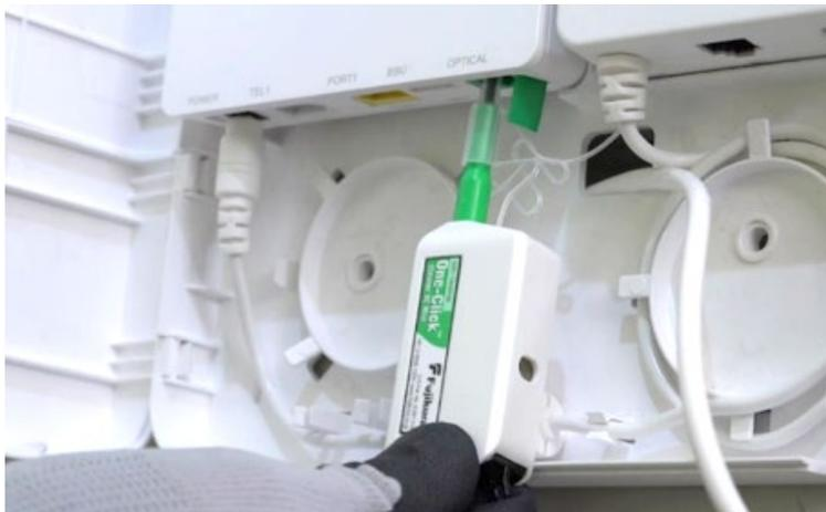
Open the green flap on the Optical port and insert the fibre cable. The cable is designed to fit only one way, so ensure the raised nodule is facing the wall when inserting.
