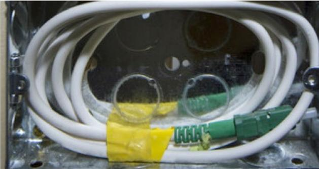
Wherever possible, the duct shall be positioned on the opposite side of the wall to where the ONT will be installed, removing the need to run internal fibre cables. However, there are cases where the kit will need to be installed away from the external lead in and your FBC will be able to advise.
