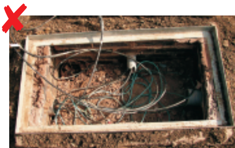
Unacceptable standard of finished box
