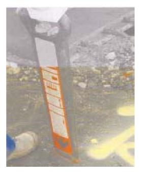
The correct size service pipe ducting must be installed at the correct depth, ensuring that sufficient room is left at each end of the duct to allow access to make the connections to the main and the service termination point. The mains connection must be left open with sufficient duct exposed to receive the service pipe and you must allow a minimum of 1m at the entry point to allow us to assemble the required fittings.
