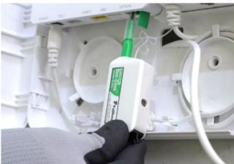
Remove the cap from the green fibre connector and use the One Click cleaner to clean both the connector and the optical port on the ONT. Once cleaned plug into the Optical port on the ONT. Care must be taken at this stage not to contaminate the end of the fibre connector to avoid any dirt from inhibiting the data signal.
