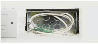
Wherever possible, the duct shall be positioned on the opposite side of the wall to where the ONT will be installed, removing the need to run internal fibre cables. However, there are cases where the kit will need to be installed away from the external lead in and your FBC will be able to advise.
